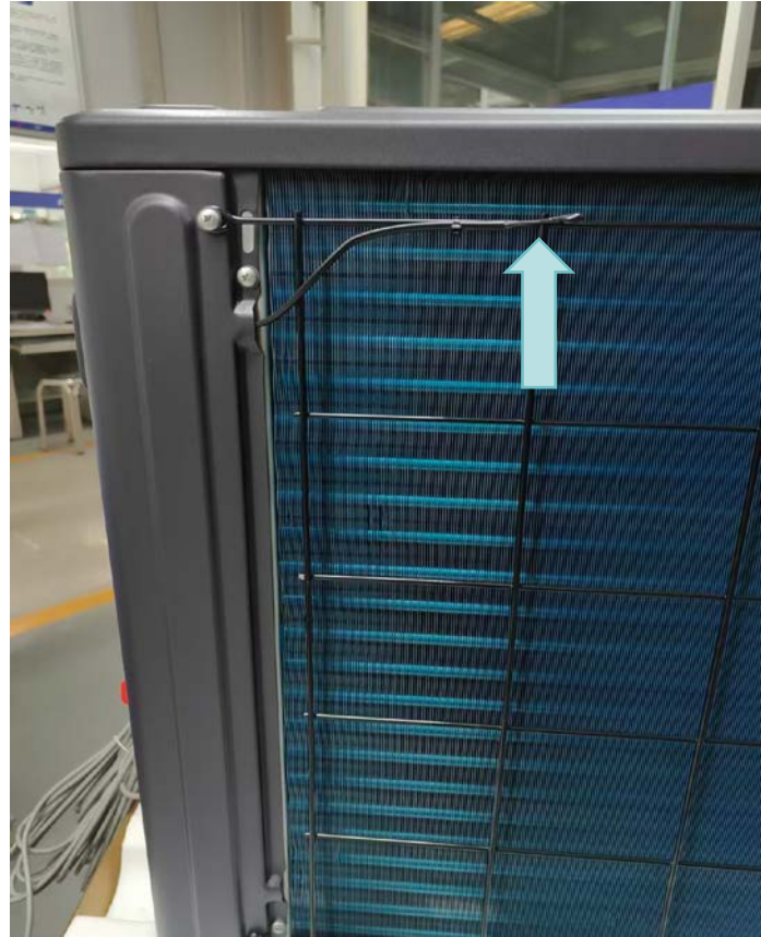
Position of the ambient temperature sensor
